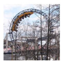
Just to the right (east) of SLÄNGGUNGAN, take the bridge over to the other side of the river and look closer at the loop of the roller coaster KANONEN (the Cannon). You may notice that the loop is not a circle, but has a larger radius of curvature at the bottom.
