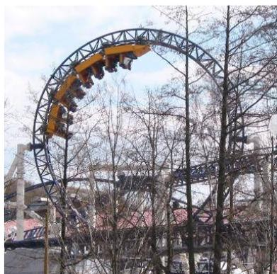
Just to the right (east) of SLÄNGGUNGAN, take the bridge over to the other side of the river and look closer at the loop of the roller coaster KANONEN (the Cannon). You may notice that the loop is not a circle, but has a larger radius of curvature at the bottom.
