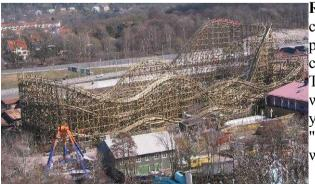
**Roller coasters** are classical examples of energy conversions, with an interplay of kinetic and potential energy as the train moves around the curves, loops, hills and valleys of the track. The Balder roller coaster was voted the best wooden coaster in the world during its opening year 2003 and also in 2005. The track has a built-in 'parabolic flight", letting the rider experience near weightlessness.
